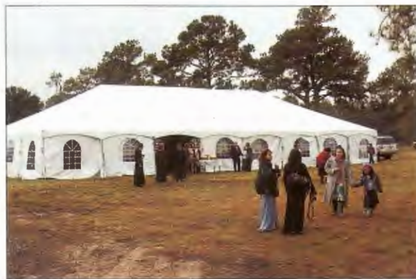
A large tent was set up on the rain-soaked property for the groundbreaking ceremony.
